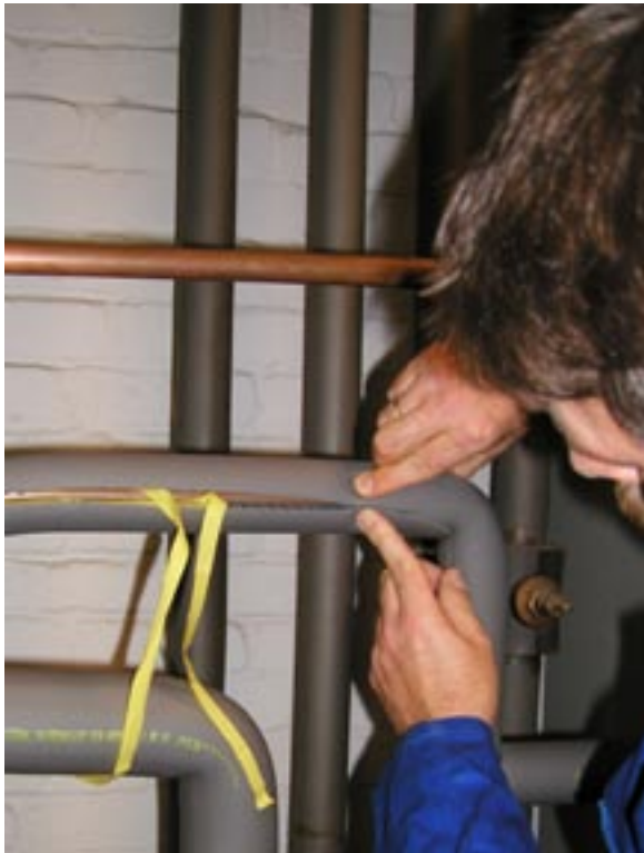
The self-adhesive SH/Armaflex tubes are ideal for retrofitting insulation to pipes: they can be installed quickly and easily even under difficult conditions on the building site
